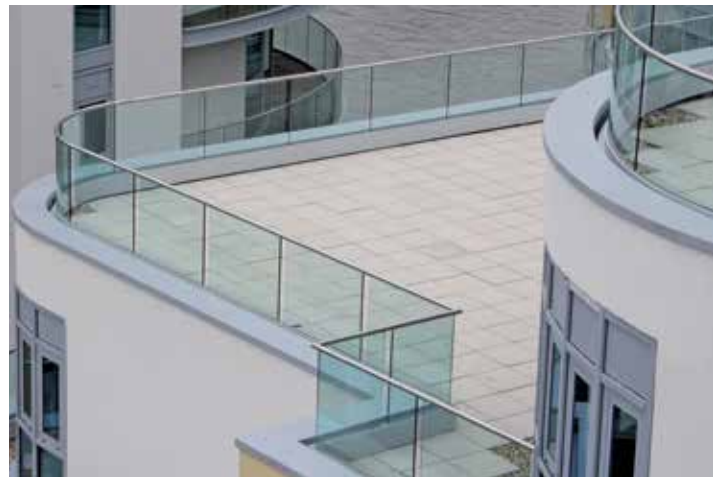
BALCONY WALL COPING
